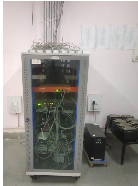
Fig. Shows Installed Fire wall
